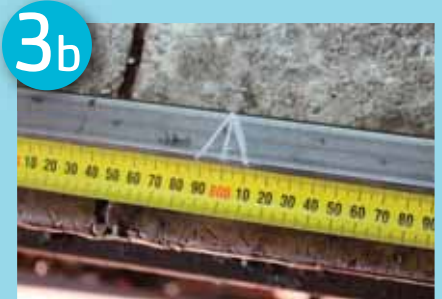
Mark 10mm on either side of the mark
