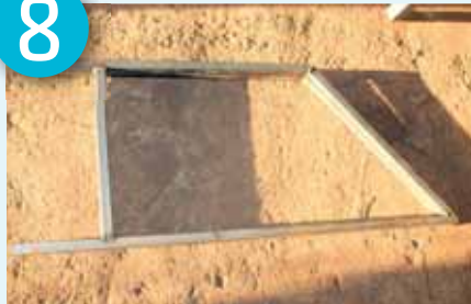
Weld cross braces in place
