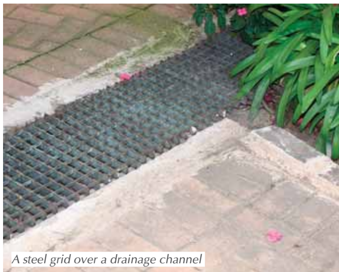
A drainage channel leading into the neighbour's garden; always check with your neighbour where the water will run
