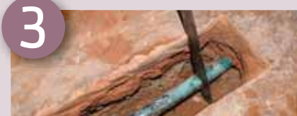
Due to the limited space we had to use a hack saw blade to cut the pipe
