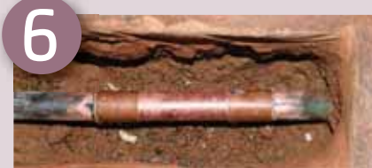
Apply soldering flux to the inside of the couplings and rotate it to transfer some flux to the pipe ends. Wipe the connections with soft tissue paper to check for water
