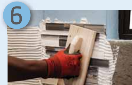
Use a grout float to embed mosaics into adhesive
