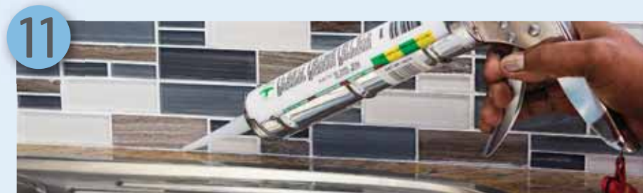
Seal the installation with a silicone sealant in the perimeter joint between the mosaics and countertop, and in any corners
