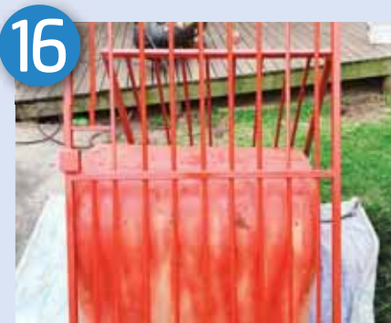
Coat with red oxide
