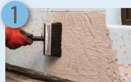
Preparation and priming
