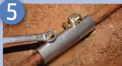
A cascade clamp can be used to seal the leaking pipe as a temporary measure
