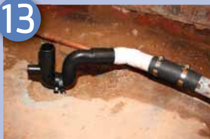
Fitting the rubber bath trap and 50mm PVC pipe with 45° elbow bend
