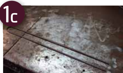
Determine the centre and bend
