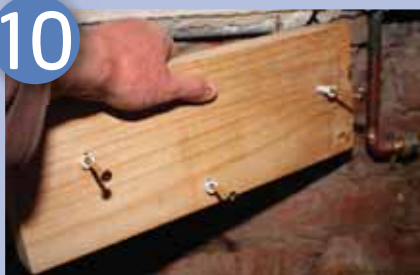
Fitting the timber support beams on the two sides which will support the bathtub at the correct level
