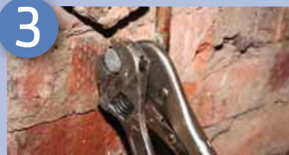
A blanking stop cap is fitted to the hot and cold-water outlets. A gas plier is used to securely hold the copper pipe while a shifting spanner is used to tighten the end cap
