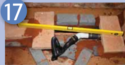
Concrete blocks were placed beneath the bathtub to protect the pipework below and the cavity filled with river sand
