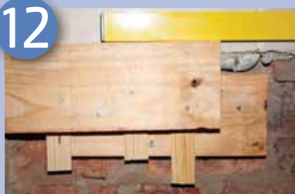
The timber support beams screwed and nailed in position
