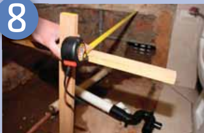
Measuring up to get the correct placement for the drainpipes
