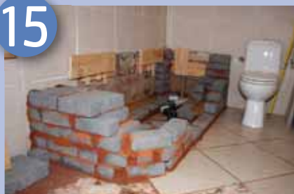
Start of the surrounding brickwork
