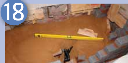
Spreading and levelling off the river sand before placing the bathtub
