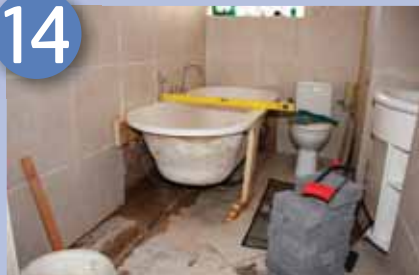
Measuring and levelling the bath
