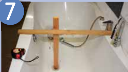
A wooden T-frame was made to measure the precise point of the drainage outlet
