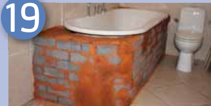
Brickwork complete with provision for a shelf at the one end
