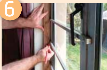
Mark discrepancies to chisel out
