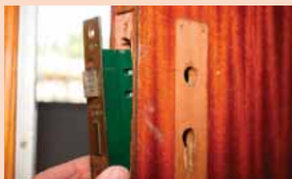
The locking mechanism must fit flush into the cavity with minimal movement
