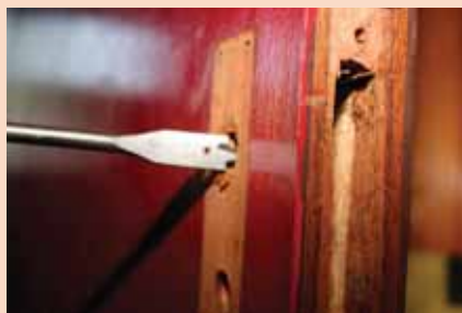
A hole-saw or auger bit can be used to make the circular holes for the key slot and spindle
