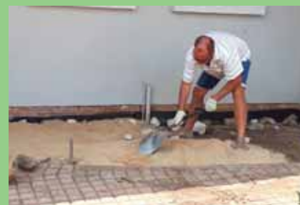
Once the dampproof lining has been laid, fill the area with river sand and compact
