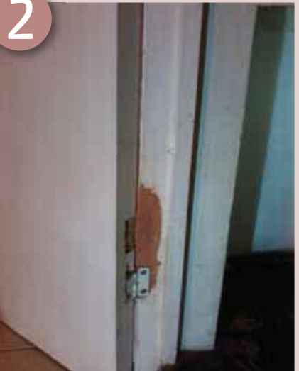
Put the door back onto the frame
