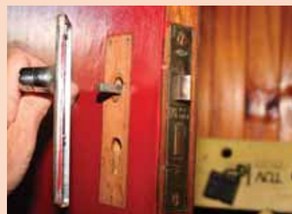
Lastly, the handles are screwed into place
