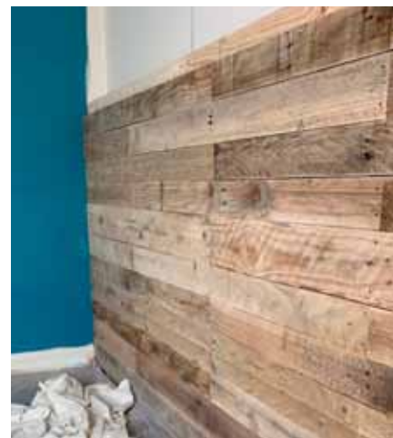
Installing the wooden panels to the frame
