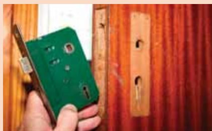
Fitting the locking mechanism
