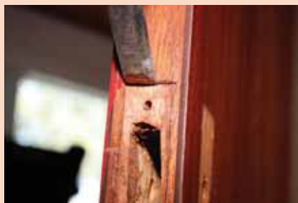
Making the recess for the lock plate
