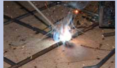
Welding thin round bar
