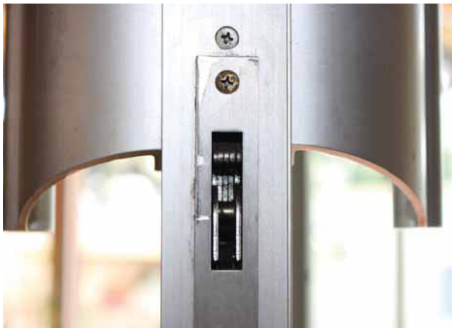
Locking mechanism for an aluminium sliding door
