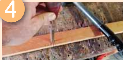
Chisel out notches for burglar guards
