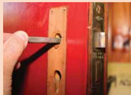
Fitting the spindle for the door handles
