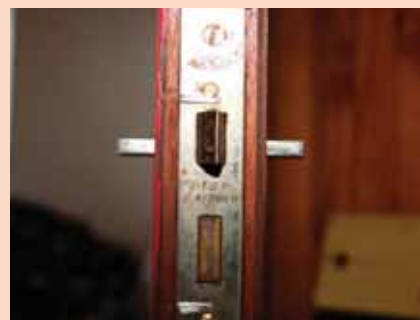
The locking mechanism and spindle firmly screwed into position
