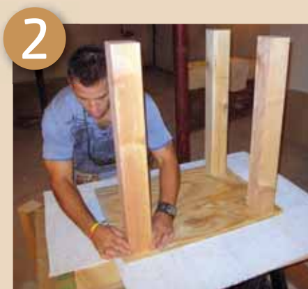
2 Position the legs on the plywood
