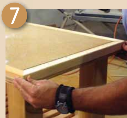
7 Frame the cutting surface
