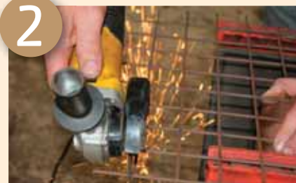
Cut the mesh to size
