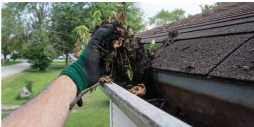
Remove debris from guttering
