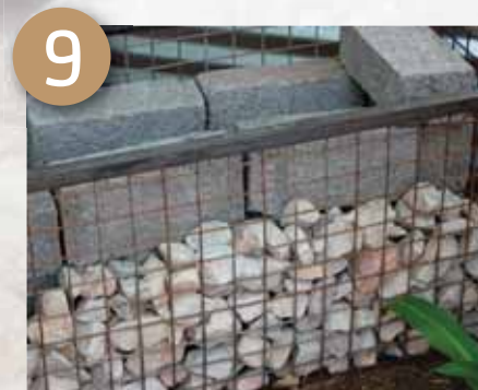
Place dump rock on the outside
