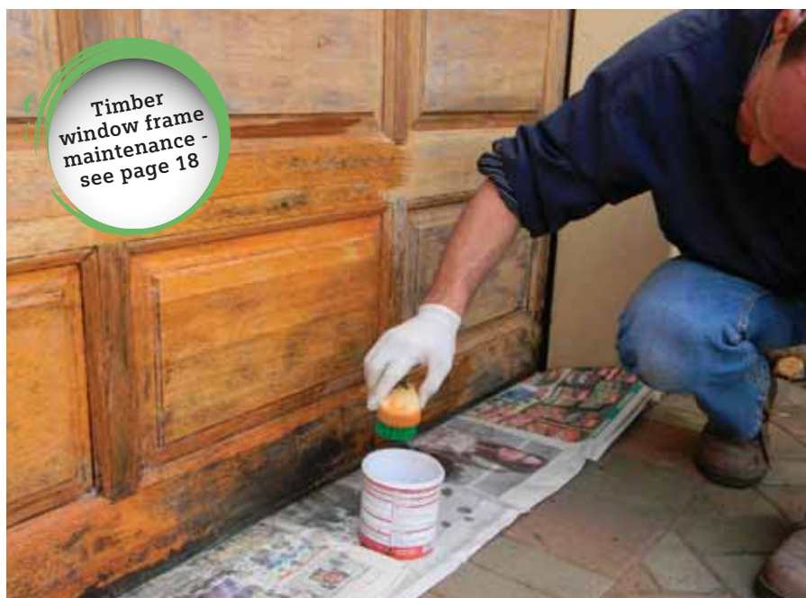
Weathered wood on garage doors must be removed before a new sealer or varnish is applied
