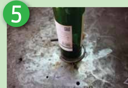
Bend the roundbar around the wine bottle
