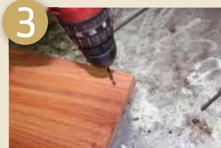
Drill the pilot holes
