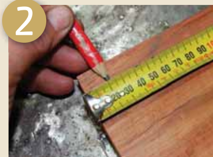
Measure for the pilot holes
