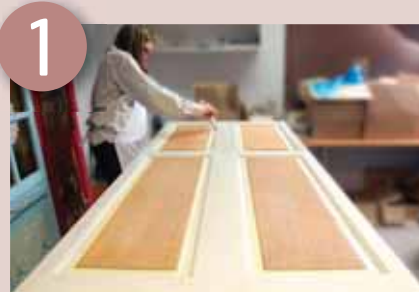
Priming around the panels
