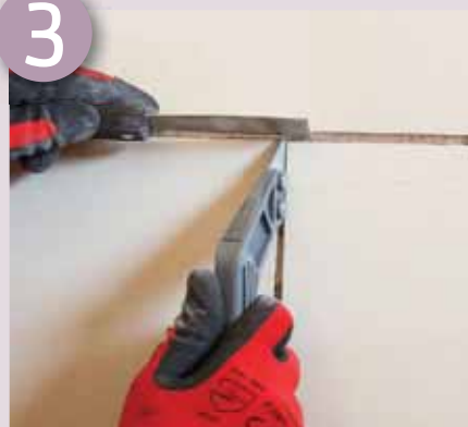
Remove existing grout
