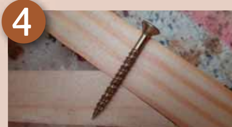
Identify the location of the screws for fixing the diagonal in place, by placing the screw in the ideal position and draw a drill guideline
