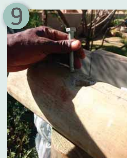
Securing the beams to the uprights
