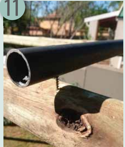
Fit steel bars to the beams
