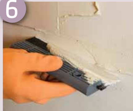
Apply the grout
