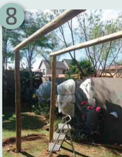
Fit the horizontal beams
